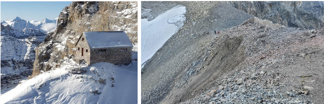
Abbot Pass Hut was built in 1922 as a shelter for mountaineers. It was substantially removed for safety in 2022 after the slope eroded underneath the structure. A selection of materials from hut were salvaged and a small ruin was left in place on Abbot Pass. © Parks Canada /D. Allen
